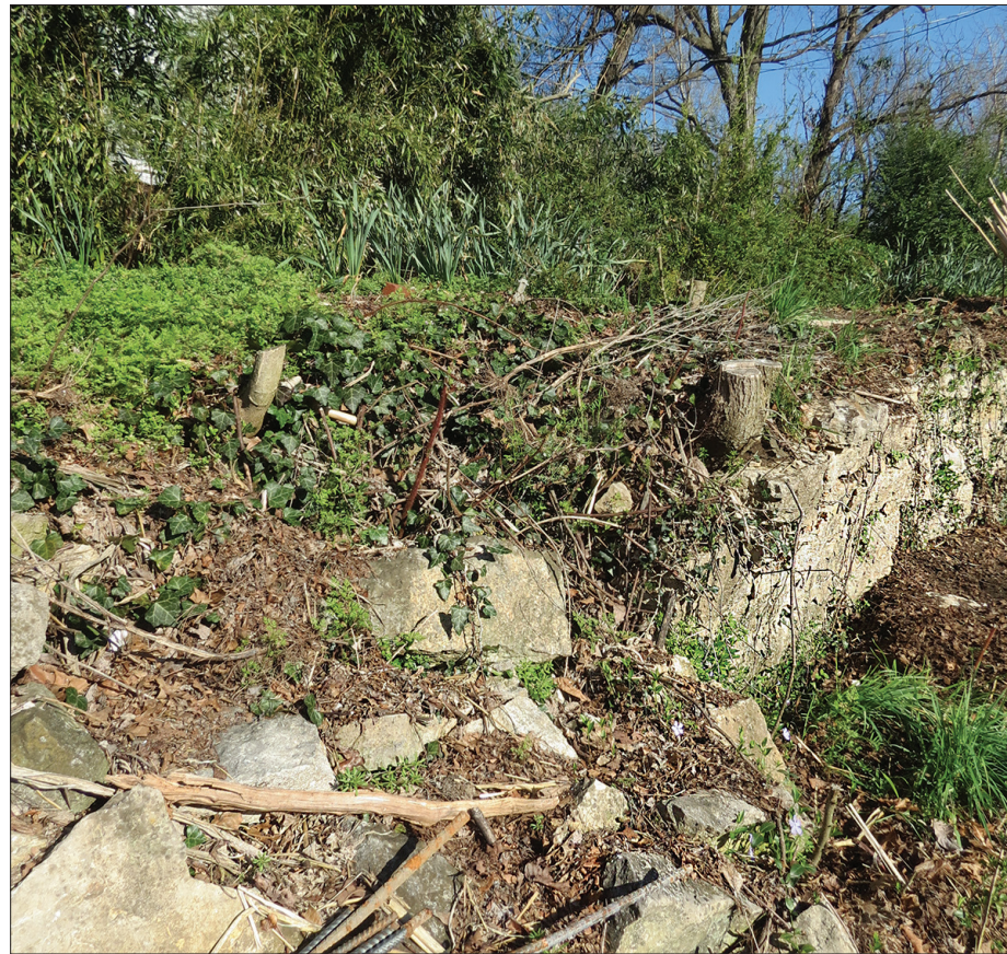
Trees should never be allowed to grow close to historic rock walls as the roots can cause failure of the rock wall as shown in the photo above. PHOTO BY BECKY GILLETTE
